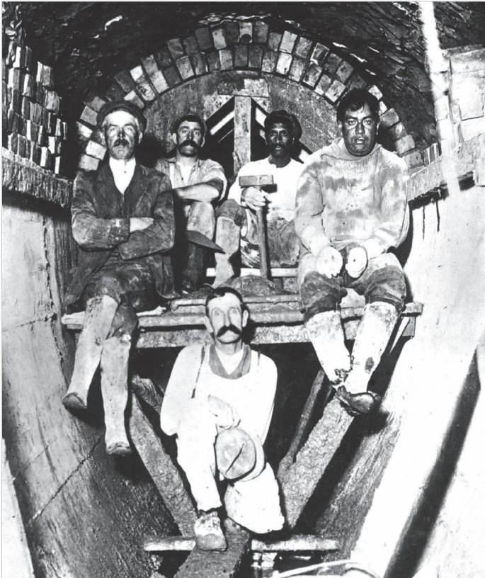
Construction workers in the first section of tunnel between Okahu Bay and Hobson Bay, 1910.
