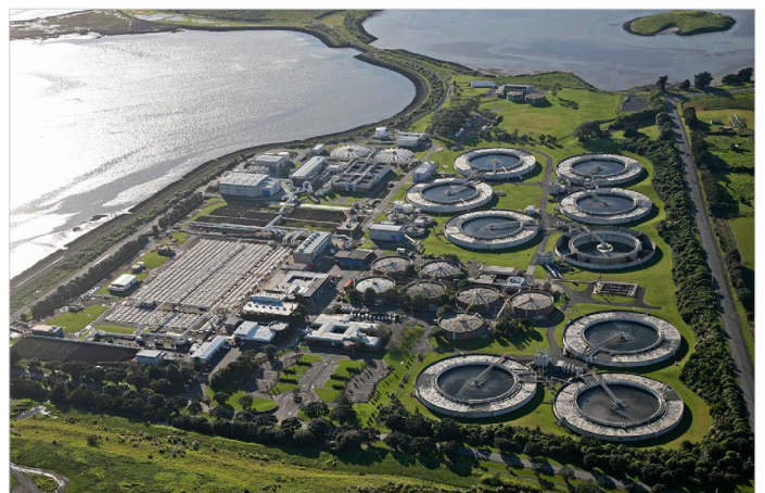
An overview of Watercare's Mangere Wastewater Treatment Plant.
